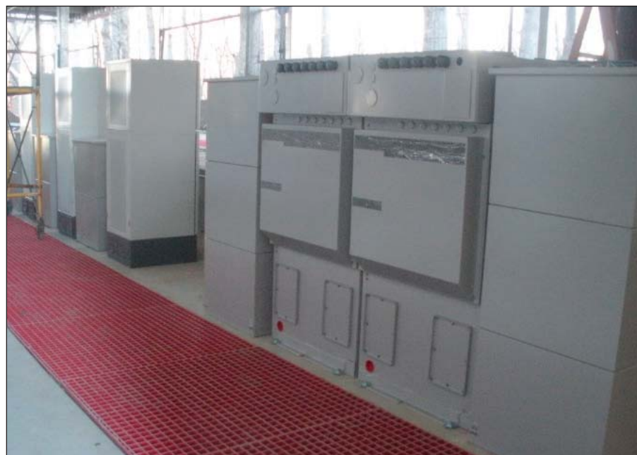
Under construction, the equipment shed for the DAS system, late winter 2014 ►
